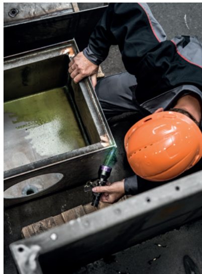
Dye penetrant testing
